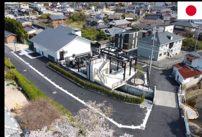
Horiuchi Pumping Station 1200mm / 2.85cms / 2.4mH / 2units 1000mm / 2.5cms / 1.9mH / 2units
