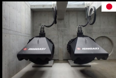
Attori Pumping Station 900mm / 1.6cms / 2.5mH / 2units
