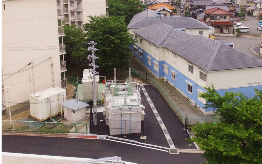
Pump Gate Overview
