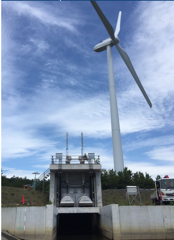
Pump Gate Overview
